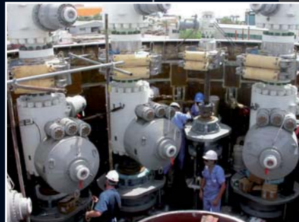
12" 2500# BALL INSTALLATION IN PROGRESS
